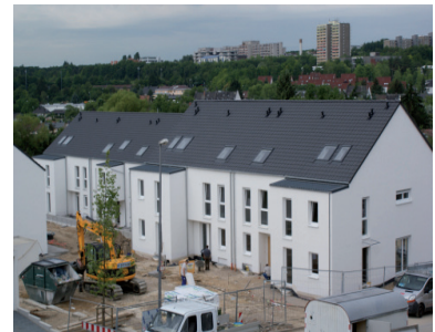
Townhouses, Wiesbaden (Germany) Planning Engineer: Wolf Joint System: wolfseal thepro® DämmDichtSystem
