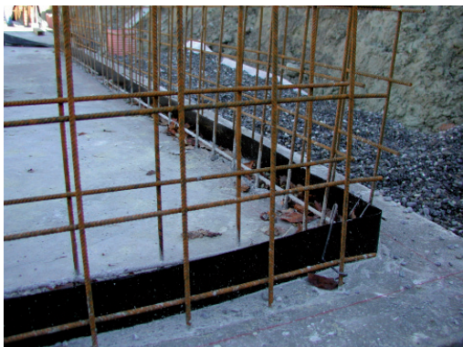
wolfseal KB joint between bottom slab and external wall
