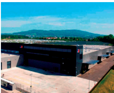
MTU Friedrichshafen (Germany) Concrete technology: Wolf
