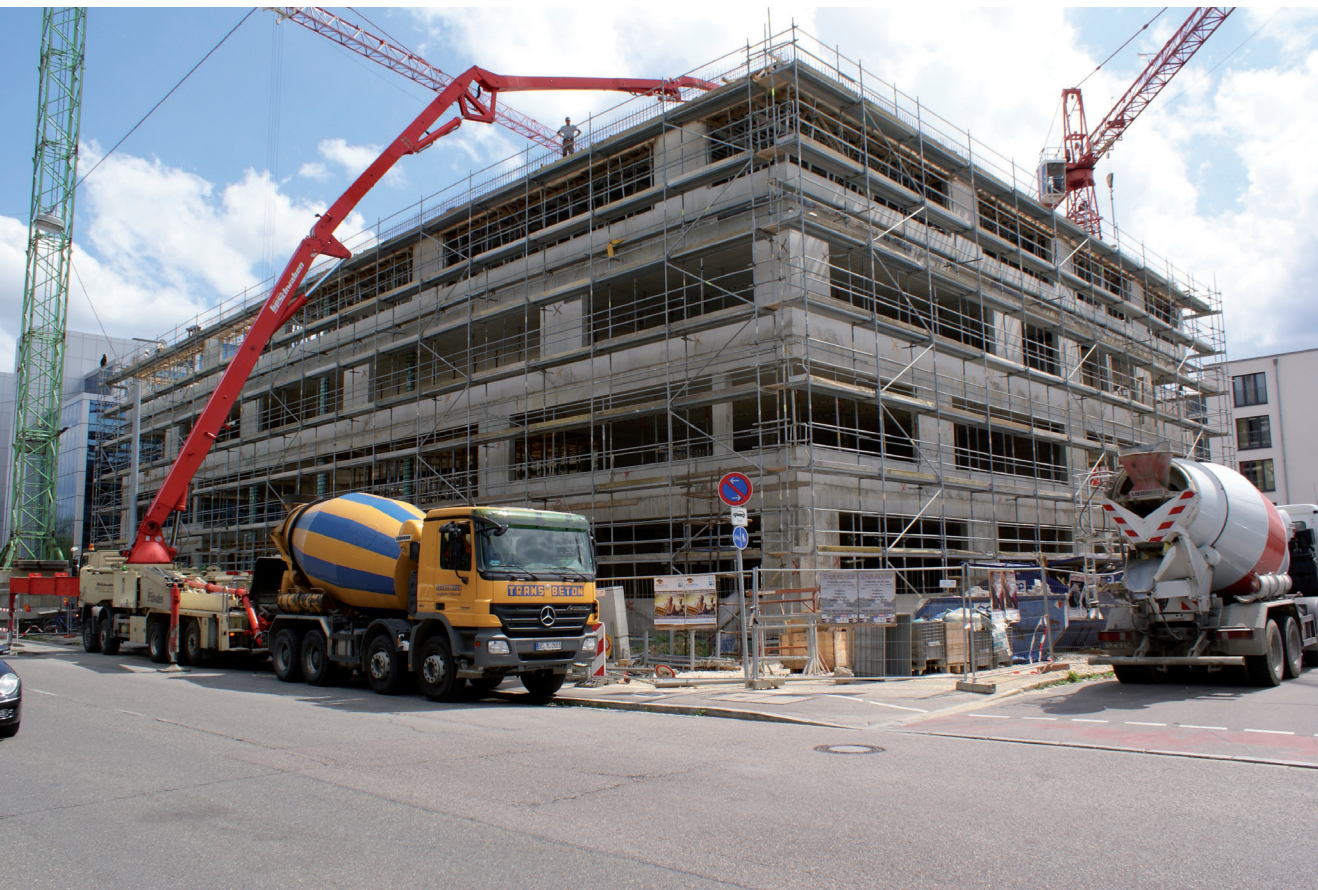
Construction site in Ulm (Germany): Using wolfseal products
