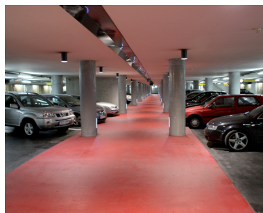
Underground Car Park, Ulm (Germany) Planning Engineer: Wolf Joint System: Pentaflex
